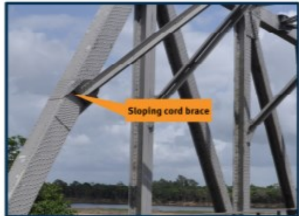
One of the sloping cord braces on the Burdekin River Bridge
